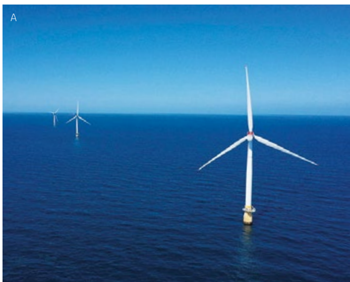
Figure 2.5 A: Hywind Scotland spar floating wind turbine; B: WindFloat Atlantic semi-submersible floating wind turbine.
